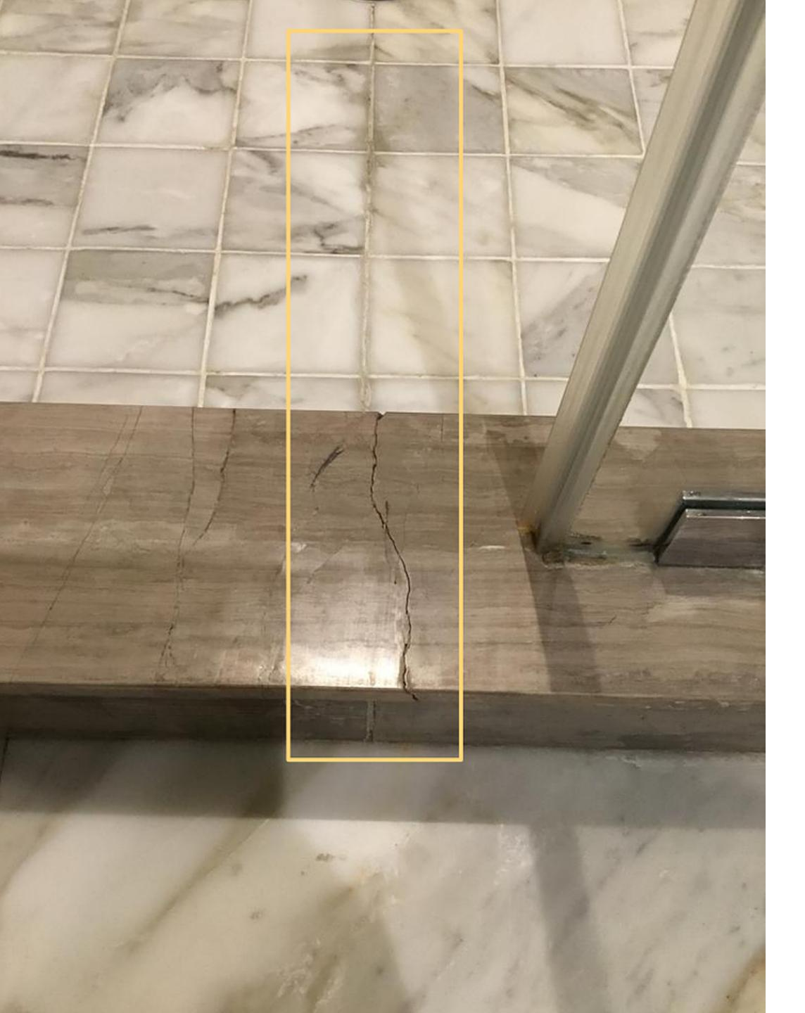
Notice the pattern where underneath moisture and water pressure has broken the grout on the floor and shower threshold leading the water and moisture outside of the shower through the substrate.
