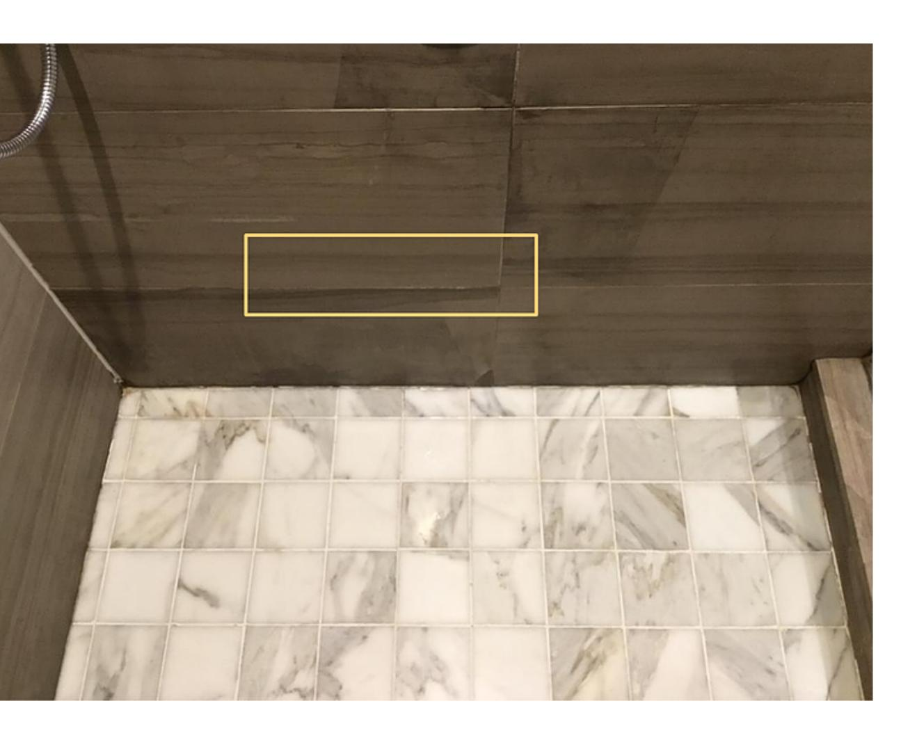
Water intrusion through grout, has already loosened, broken and shifted some of the marble tiles.
