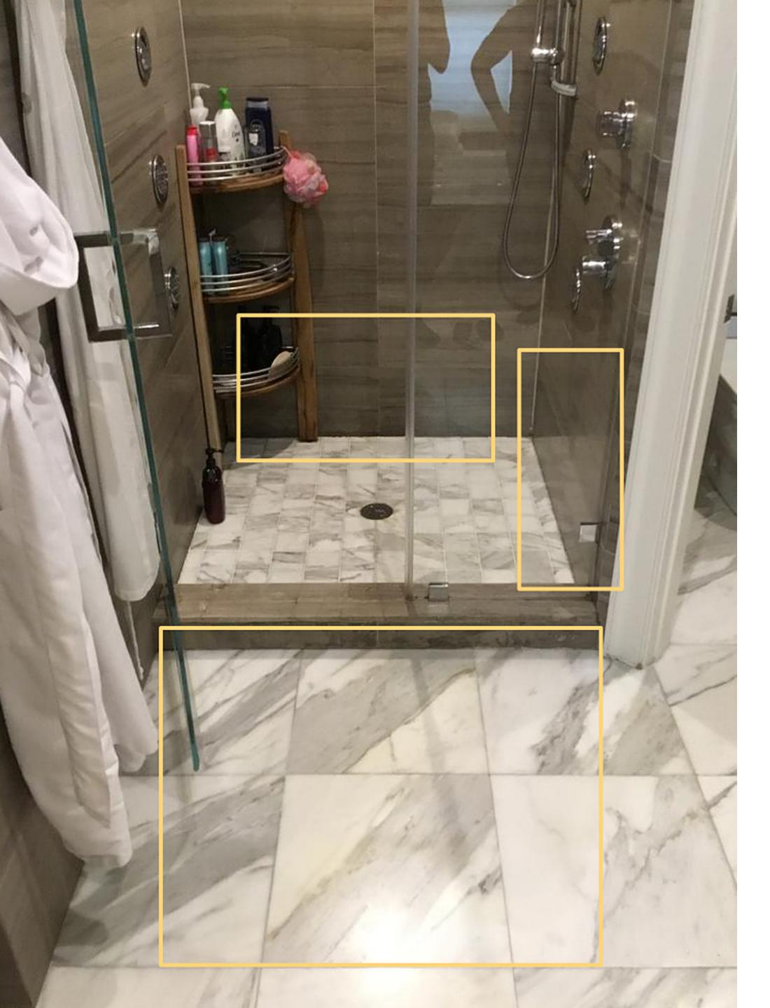
Water and moisture has raised up and out of the shower, about two feet outside the shower floor substrate. Not visible on the surface.
